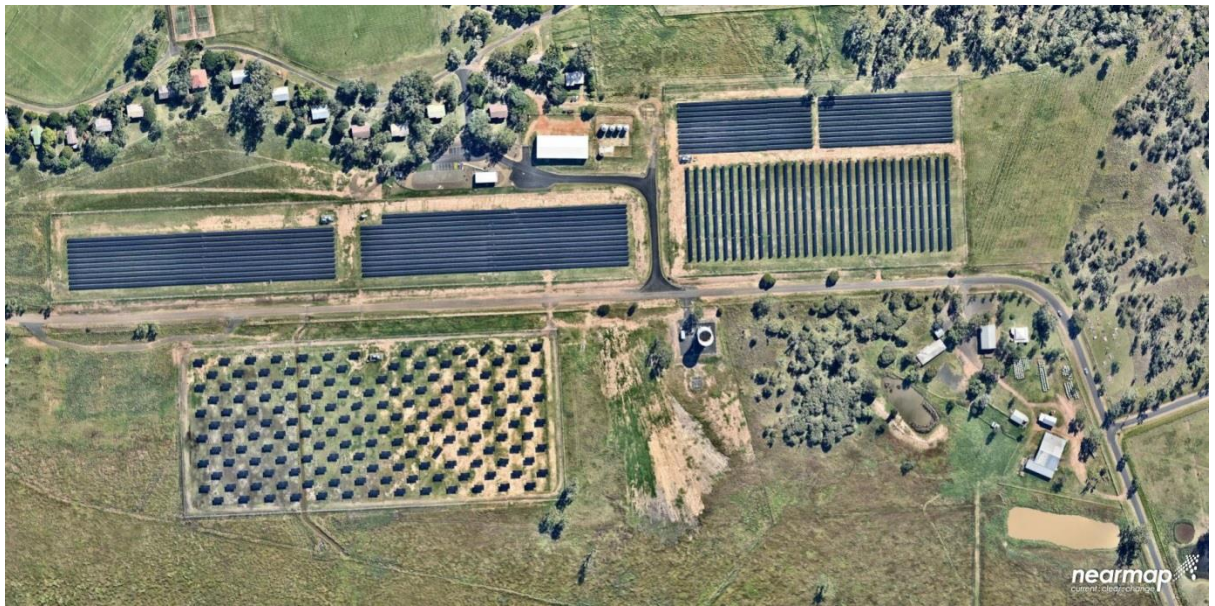
Figure 1. NearMap Picture of the GSRF Solar Array
